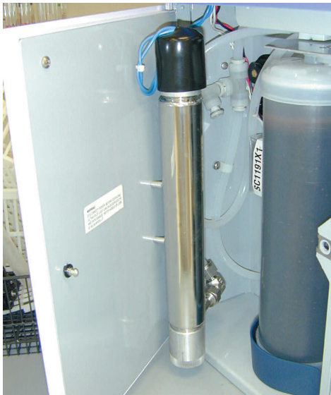
Figure 1: UV Lamp Installation - Left side view
